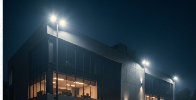
Perimeter & security lighting
