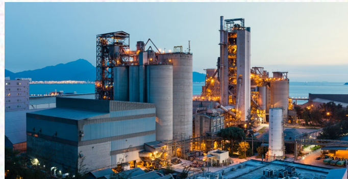
Industrial & material handling areas
